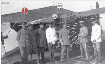
Rear view of the same aircraft shown above thought to be 5685/17. The top surface of the wings are covered with light 5 colour pre-printed lozenge fabric applied at a 45 degree angle. The cross fields seen here are noteworthy because this white square was superseded by a 5cm outline in November 1916. It is unlikely these were incorrectly applied at the Halberstadt factory and it is thought that some units backdated the newer markings either as a form of unit identification or to try and fool the enemy that they were flying in older, outdated equipment.
